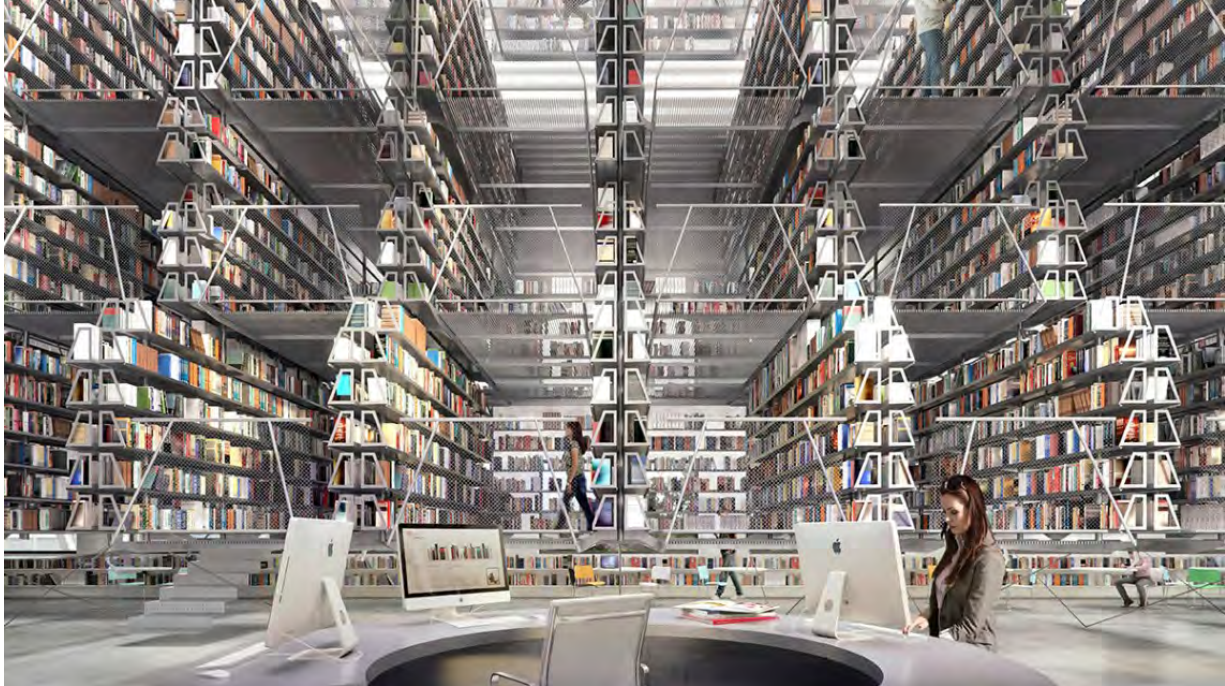
Figure 12. Renderings provided by the architect show perforated floor panels that violate basic principles of compartmentation by connecting more than two stories; larger “6-inch flue” openings also appear in each story under the bookstacks.
